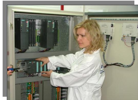
Fig. 1: Full CPU redundancy with 2 Simatic S7-412 PLC's.
